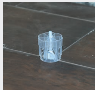
Linear leveler installation.
