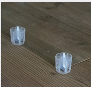
T-shaped leveler installation.
